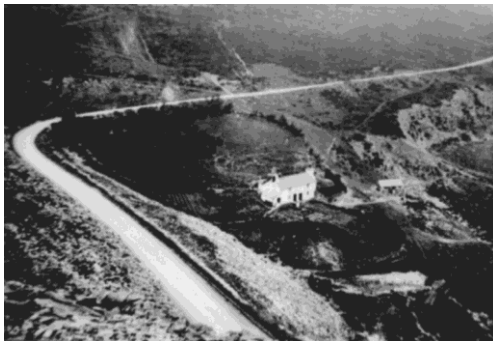
This photograph from around 1900 clearly shows Tŷ Issa as two cottages.
