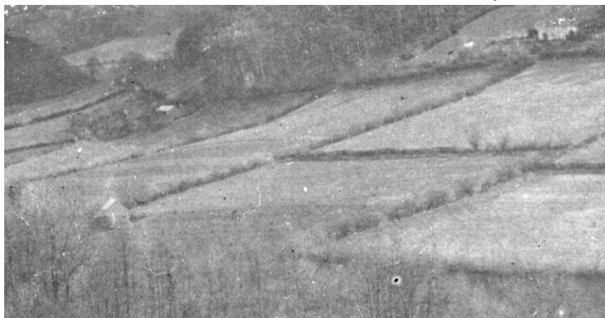
A photograph from the 1930s or 1940s. In the top right corner of the photograph can be seen Birch Cottage and, towards the bottom left, the building of Tŷ Isaf.
