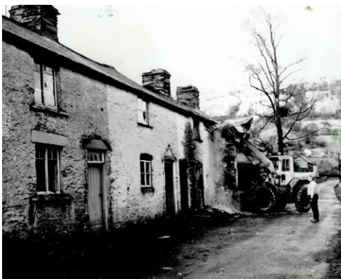
The demolition of Post Office Terrace.
