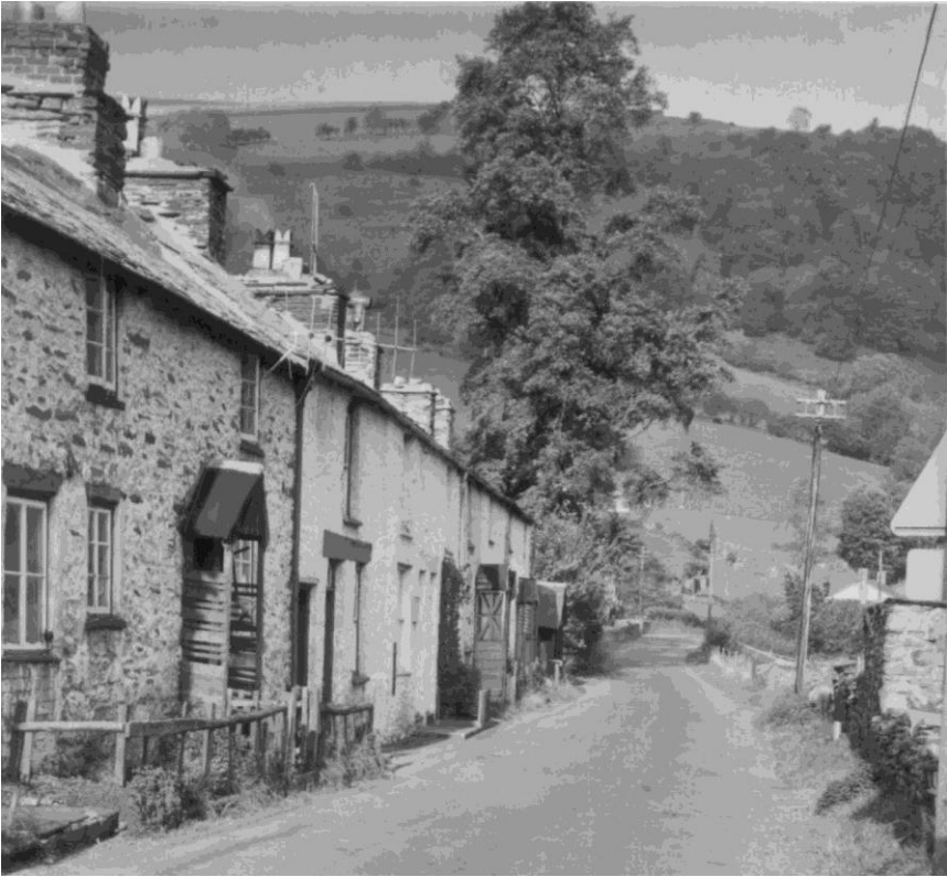
Post Office Terrace. The Post Office is the third house in from the left, with the post box set into the wall next to the window. The rough rubble construction can be seen in the nearest cottage.
