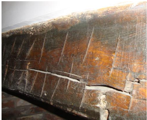
The beam over the inglenook fireplace showing the adze marks
