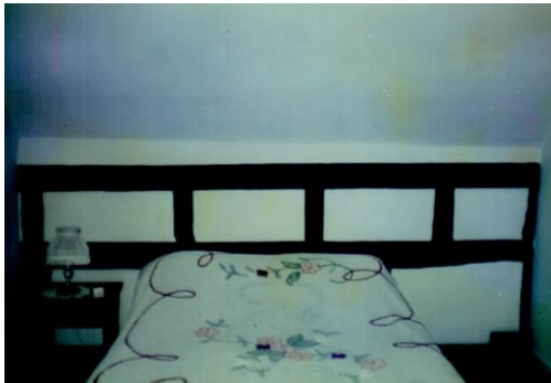
The timber framing exposed inside Pentredŵr Farm.
