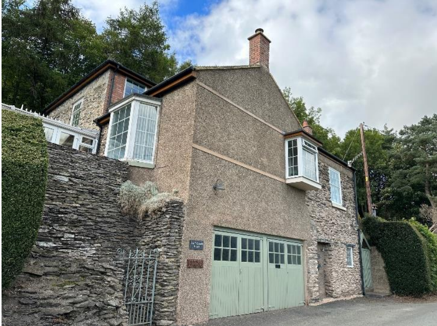
The front elevation of Pen y Clawdd House in 2023.
