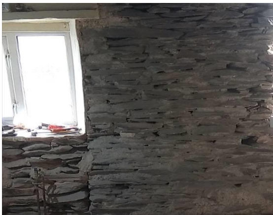
Plaster removed from the interior walls.
