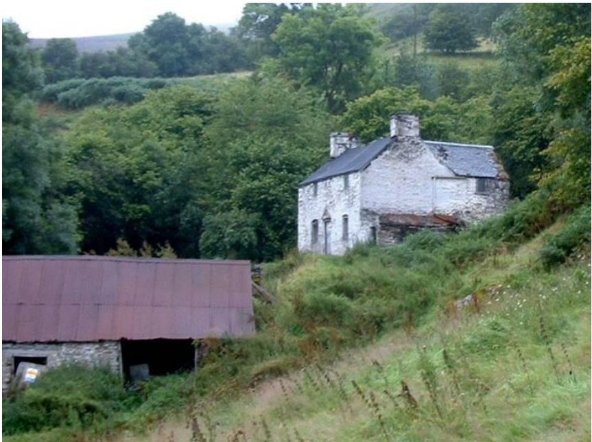
The dilapidated original building of Oernant Isaf in 2007.
